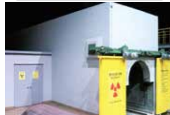
RT bunker & lead door with safety system
